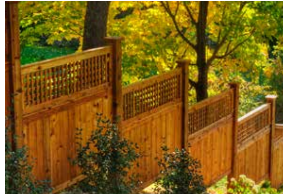
A recent installation of a western red cedar courtyard fence by Atlas Fence.
